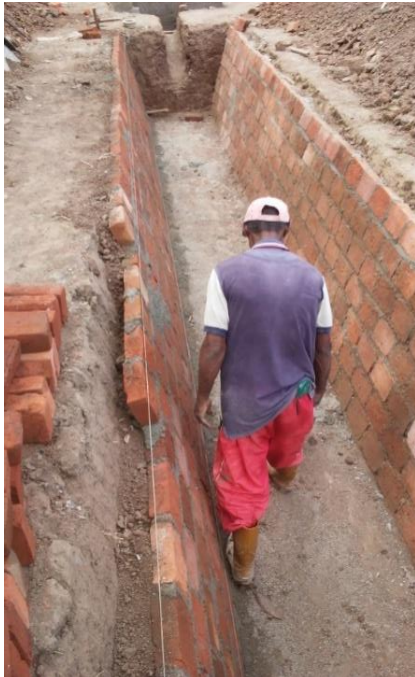
Photo 2. Trench lining process in preparation for the installation of a biodigester at the Julio Trigo Credit and Services Cooperative.
