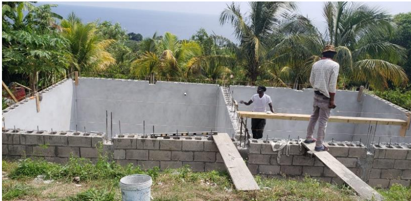
Photo 3: Construction of water catchment
