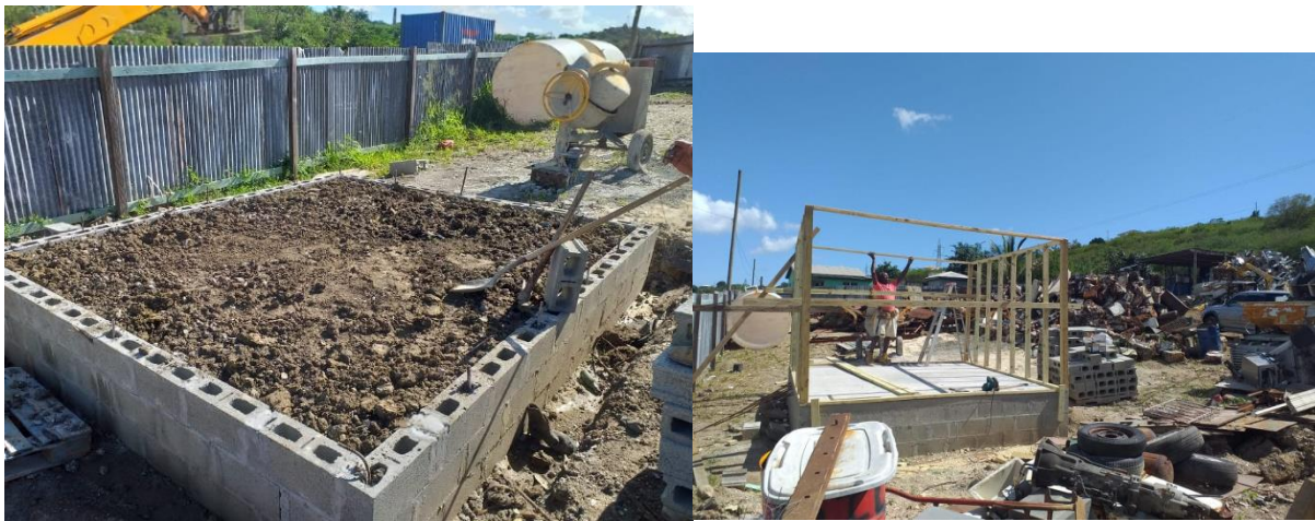
Photo 2. Construction of wire stripping center to house equipment
